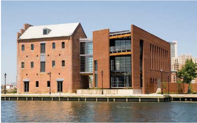
Photo 1 Reused (left) and New Brick Buildings
